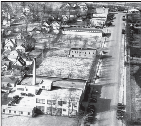
Main Street looking north from 12th Street. Allison Plant No. 1 in foreground, 1925.
